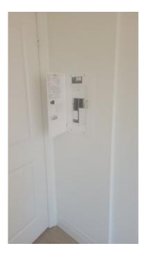
Panel Amperage Rating The electrical capacity of main breaker was listed / labeled as 125 amps.
